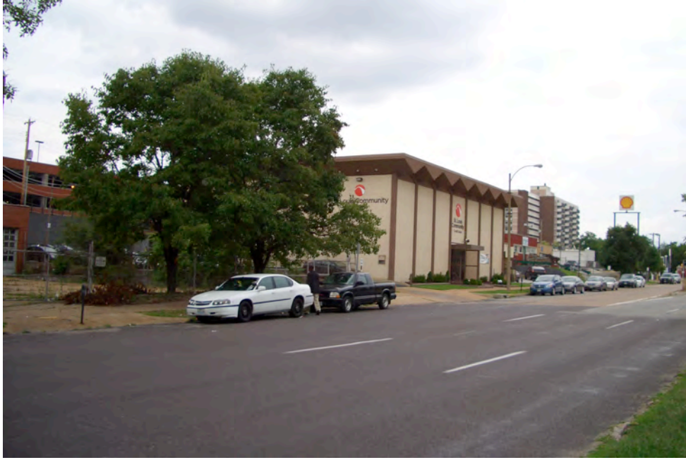
Buildings Adjacent To 3663 Forest Park Avenue To The East
